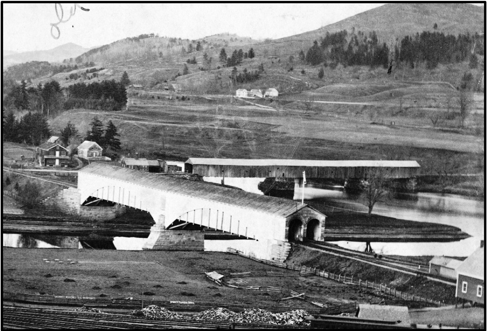
The Connecticut & Passumpsic Rivers Railroad bridge over the White River at White River Junction, Vermont. A Massive Burr Truss two-track wooden bridge built in 1848.
