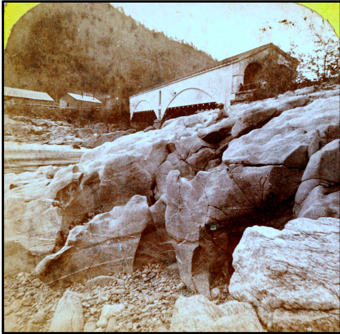
The Cheshire Railroad bridge at Bellows Falls erected in 1849. A Burr Truss type of wooden bridge.
